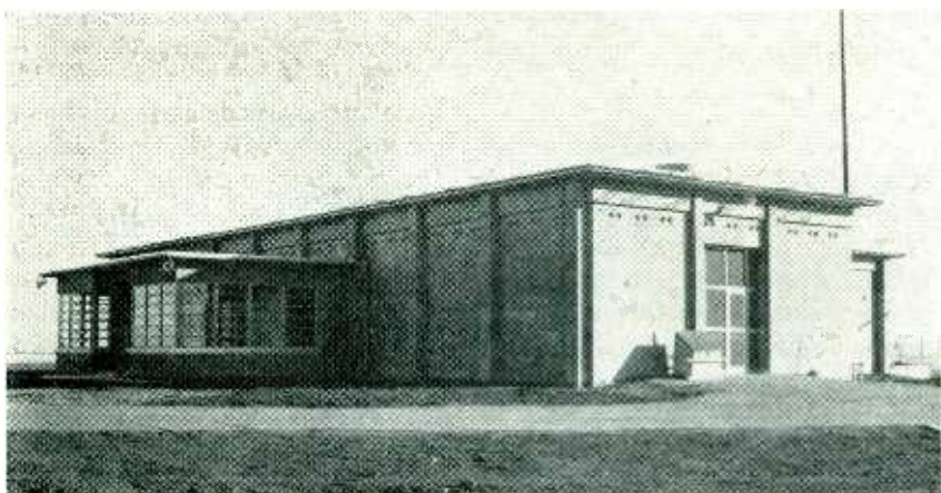
Exterior of Dixon, California station. Holes under cornice are for feeders
