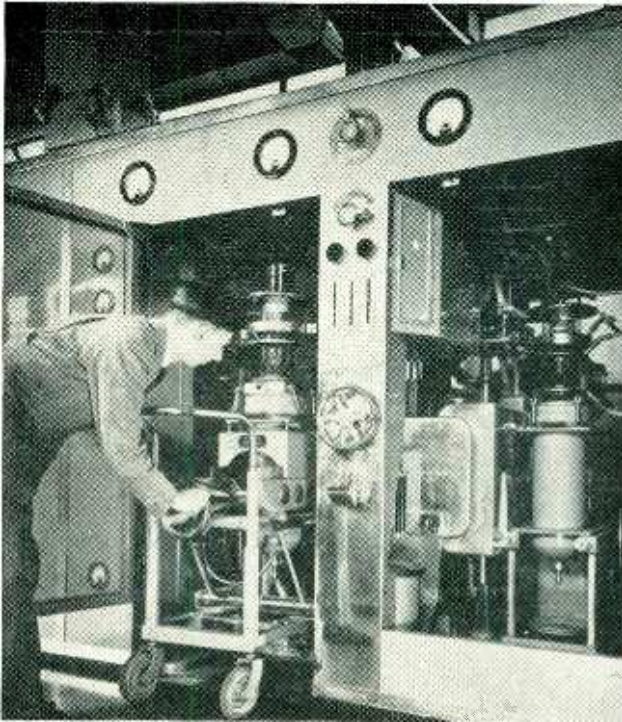
Changing a 50-kw tube in EBC final amplifier. Dolly speeds work and avoids damage to equipment
